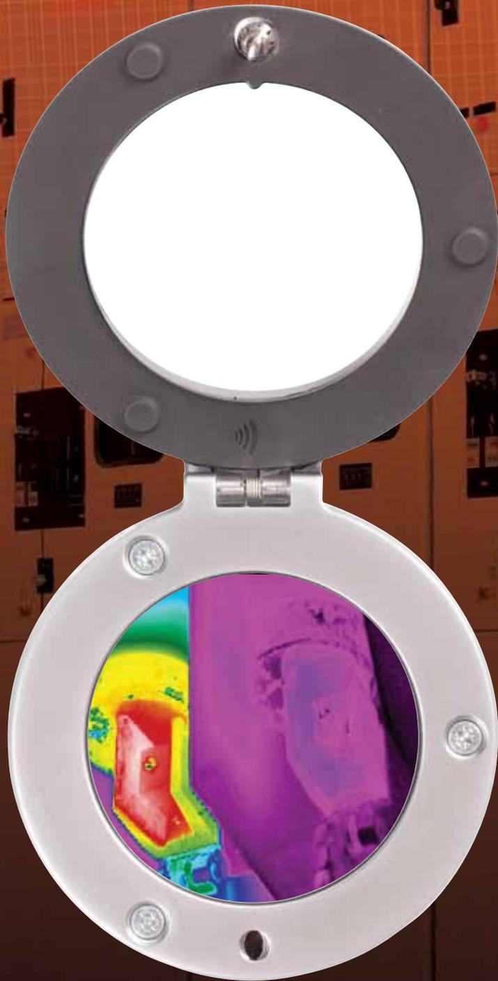
“Installing Intelligent IR Windows is a cost effective method for performing thermal surveys in accordance with NFPA70E requirements.”
